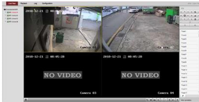
Fig.3. Access and control of the CCTV system
